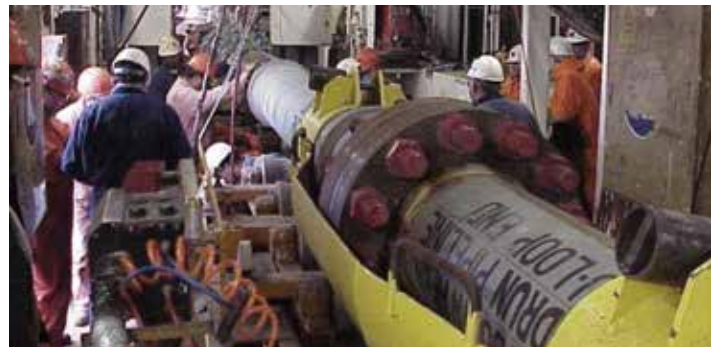
S-Lay Installation
