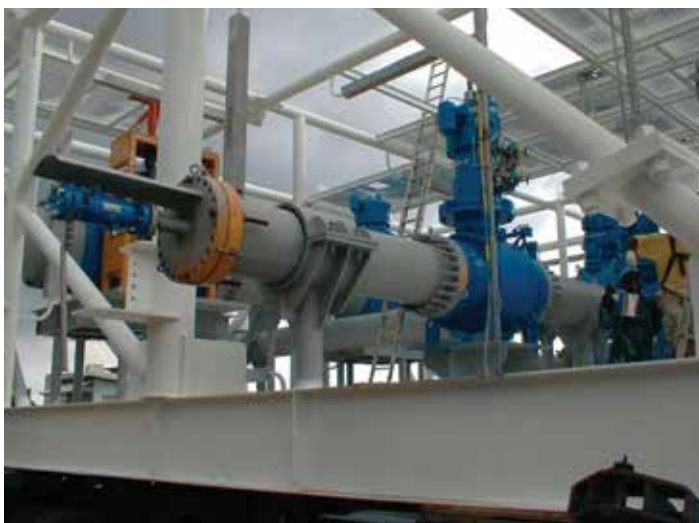
Taper-Lok connector on 26 inch Subsea Ball Valve
