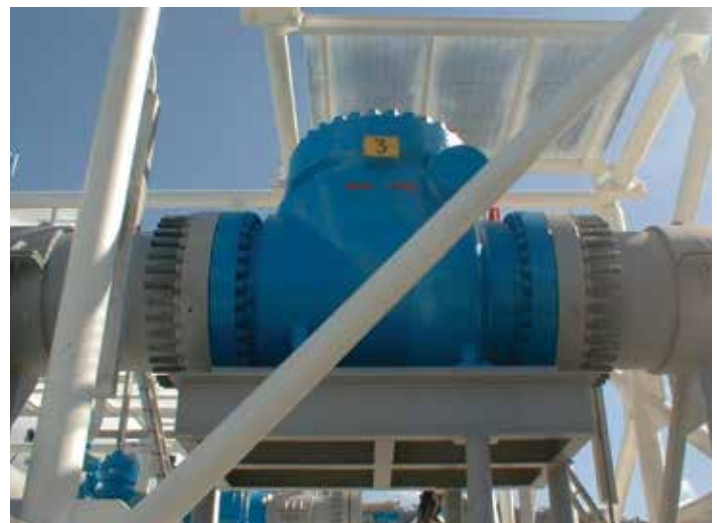
Taper-Lok connector on 48 inch Subsea Check Valve
