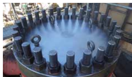
Taper-Lok Retrofit Complete
