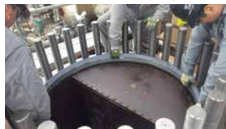
Install Taper-Lok Seal Ring
