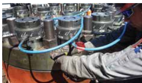
Tensioning the connection
