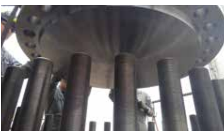
Install Taper-Lok male blind cover flange
