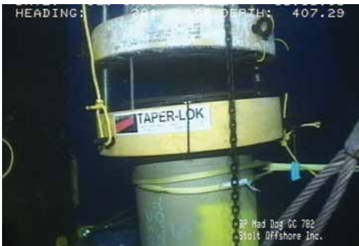
Diver Installed Riser
