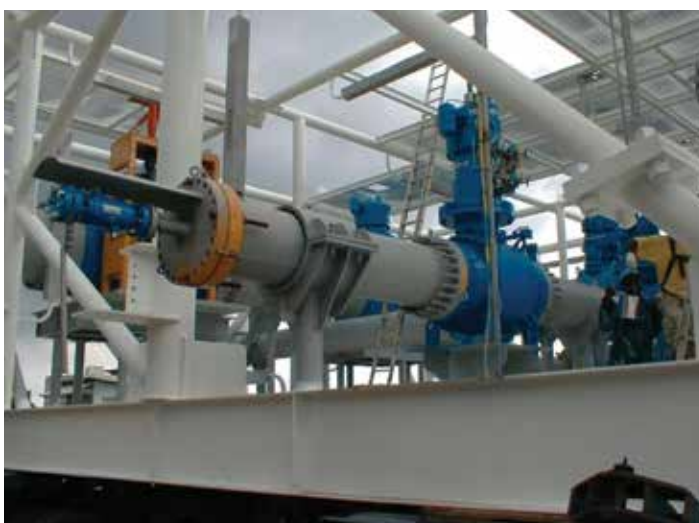
Taper-Lok® on 26 inch Subsea Ball Valve
