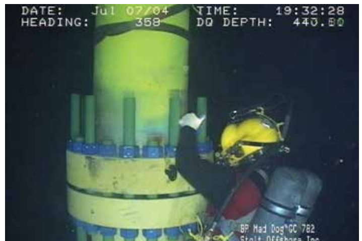
Diver Installed Riser
