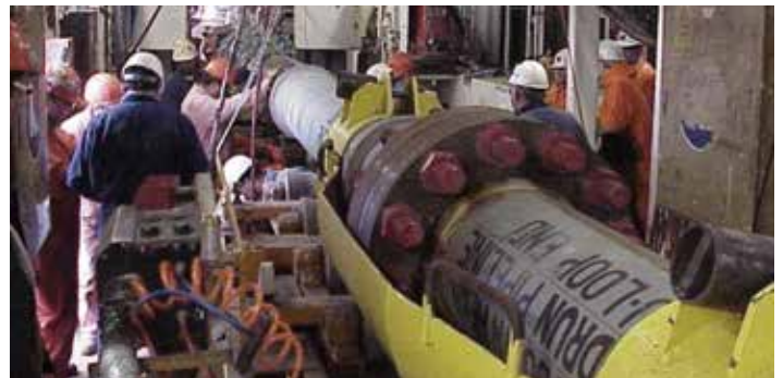
S-Lay Installation
