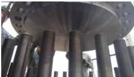
Install Taper-Lok male blind cover flange
