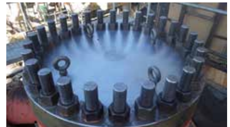
Taper-Lok Retrofit Complete
