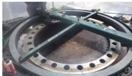
Machine Taper-Lok female seal groove into existing exchanger channel
