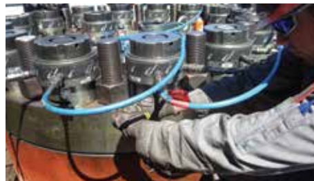
Tensioning the connection
